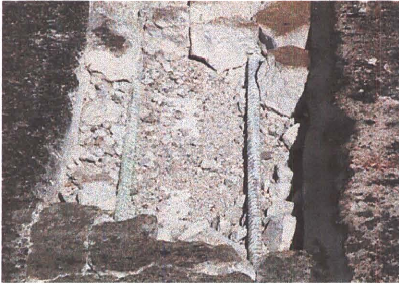
POT HOLE WITH EXPOSED REBAR AT "A" APPROACH
