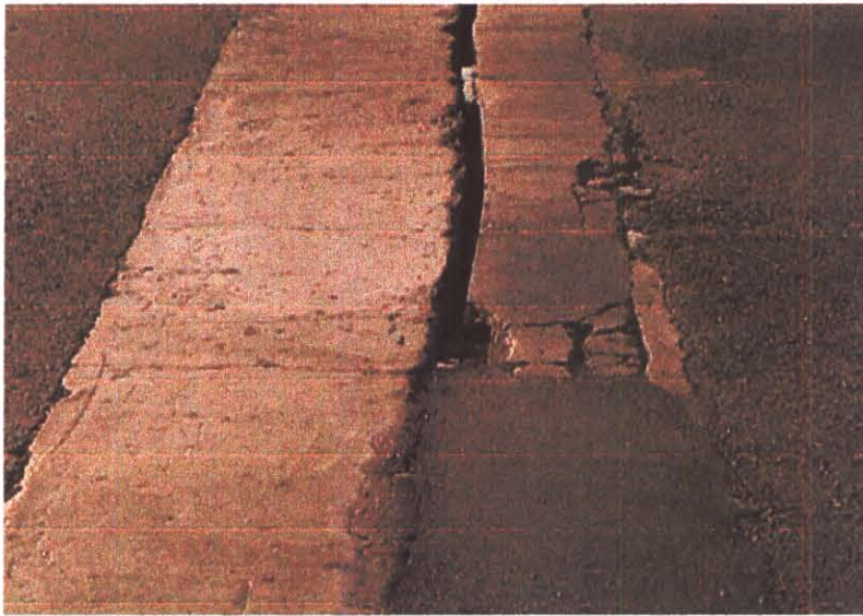
EXPANSION JOINT AT "A" END MISSING FILLER
